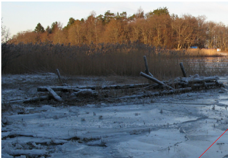
Bryggan innan renovering.
